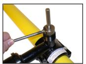
15 To allow flow through service, back punch up until the top of the punch is flush with top of saddle. It is important that the punch does not protrude above the top of the saddle tee.
