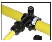
16 Verify that the O-ring is in the cap. Install cap on saddle hand tight. Do not use wrenches on cap.
