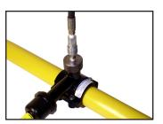
13 Remove cap, then insert drive key (use drive key 33-5505-00) into punch.
