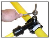
14 Screw punch down until stop on drive key contacts the top of the saddle tee. The tap is now complete.
